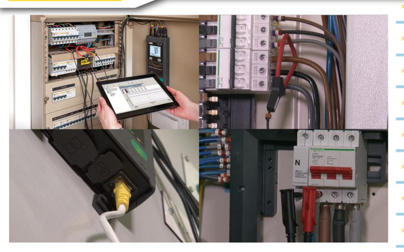
These PELs can be self-powered from the installation to which they are connected, and plugged into the computer network for remote monitoring. Or just interrogated regularly through a tablet or smartphone.
