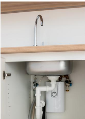
In terms of energy consumption, zooming into the 1 second sample logs it could be seen that the old heater came on for approximately 3 minutes every 140 minutes as it strove to keep the water inside at the set temperature. During these 3-minute periods it drew 2,192W and this occurred 10 times per 24-hour period. A total of 30 minutes per day at 2,192W equalling 1,096Wh, essentially 1KWh.
