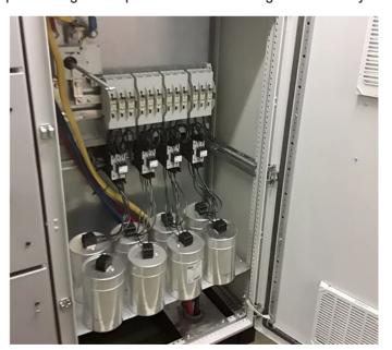
Selection of the correct design of power factor correction is critical to ensure long term reliable operation of a facility. With the increasing use of non-linear loads in industry, such as variable speed drives, LED lighting, large quantities of IT equipment, etc. and their associated harmonics, it may be the case that none of the traditional methods discussed so far for power factor correction will be suitable.
