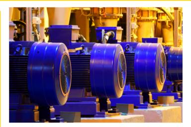
motor (apparent power) is made up of two components: active power and reactive power. You pay for both, but only the real power does useful work. The ratio of the active power to the apparent power is known as the power factor, and the nearer this is to 1.0, the less money you're spending on useless reactive power.
